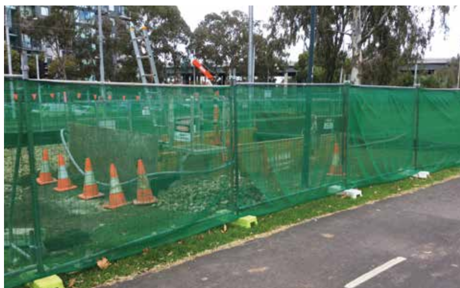
The launch shaft set up with a Davit Arm.
