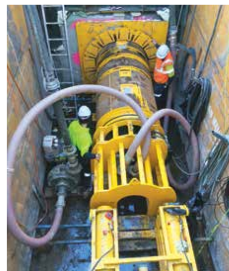
The launch of a TCC 900 closed face tunnelling machine.
