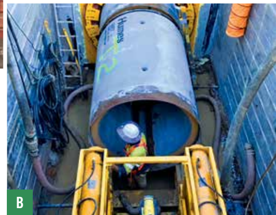
A: D.J. Mac Cormick's MTBM being lowered into the launch shaft.
