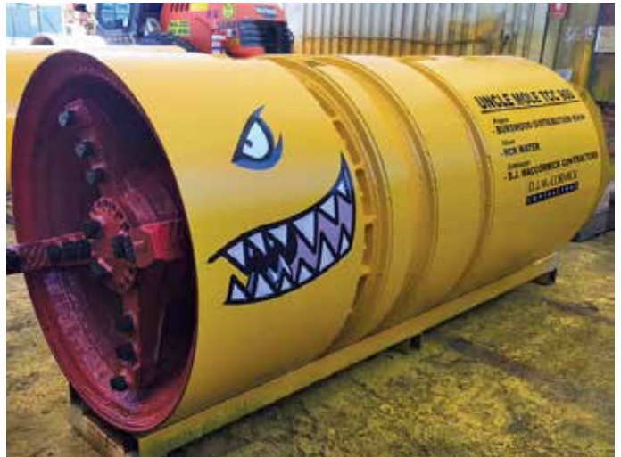
The project TBM on site.
