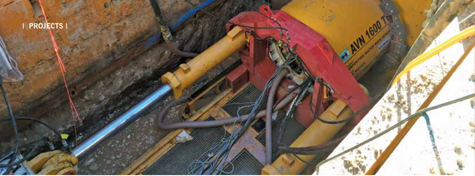
Launching the Herreknecht AVN 1600 microtunnel boring machine.
